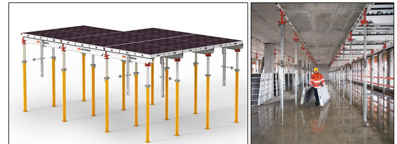
Skydeck system (left) and decking panels removed with back propping left in place (right)
