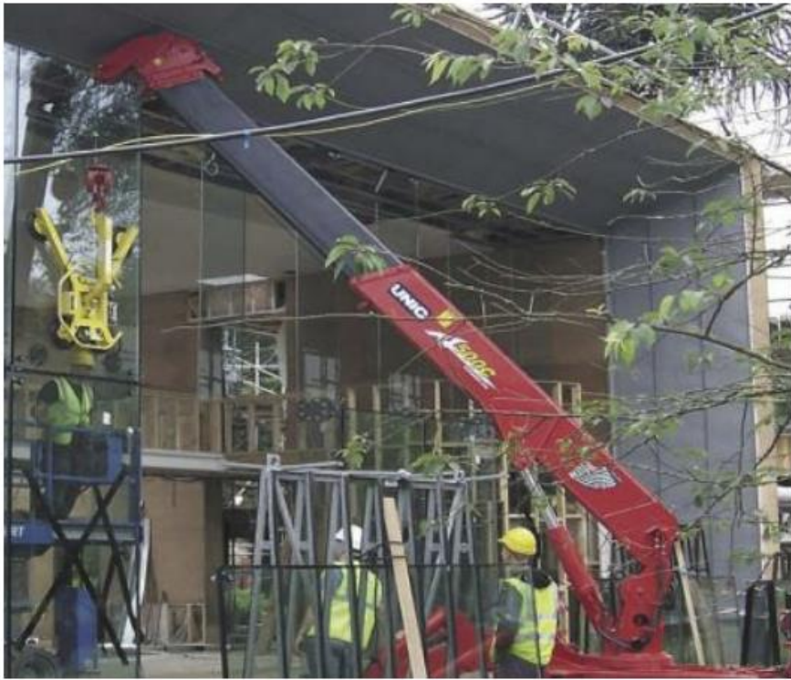
Installing ground floor glazing using mini crane and power sucker.
