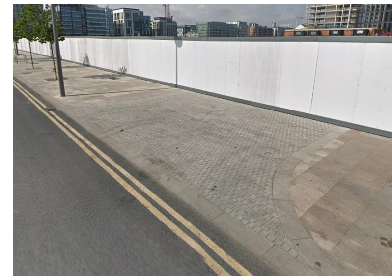
Existing Dished Footpath on North Wall Avenue Proposed for Use as Main Vehicle Entrance
