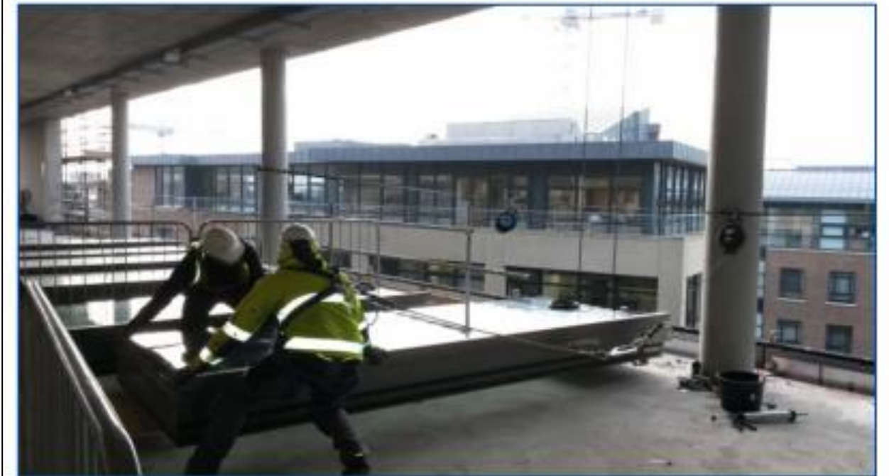
Crane lifting from floor above
