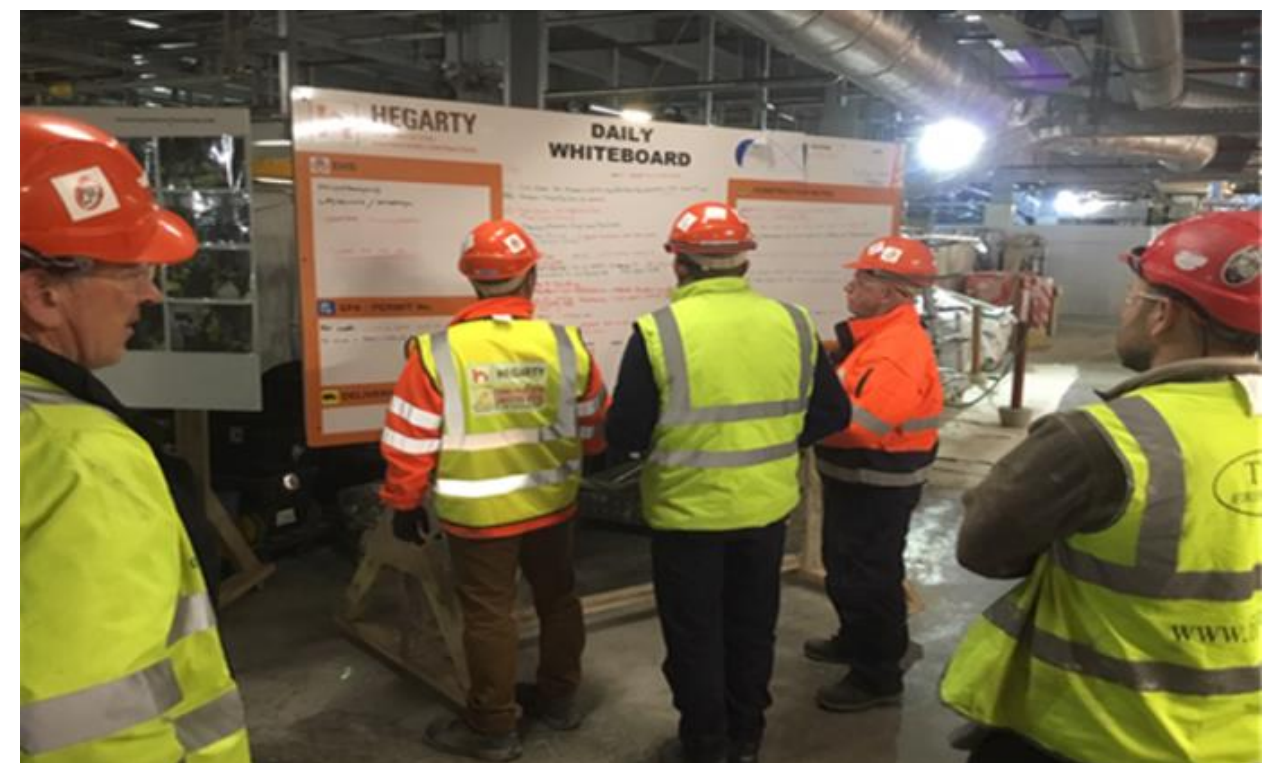
Daily Whiteboard Meeting – Attended by Project Manager, Area Supervisor and Subcontractor Foremen
